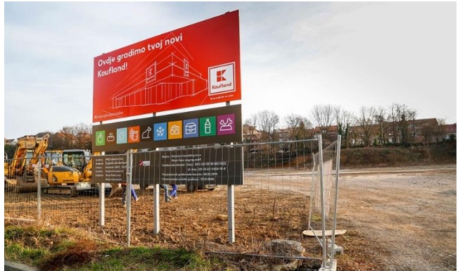
Figure 7: Kaufland construction site
