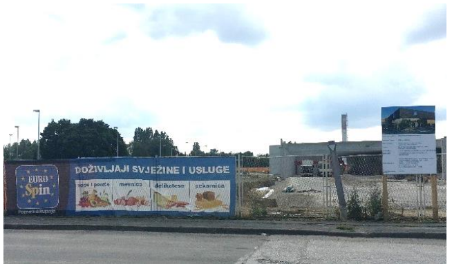
Figure 8: Eurospin construction site
